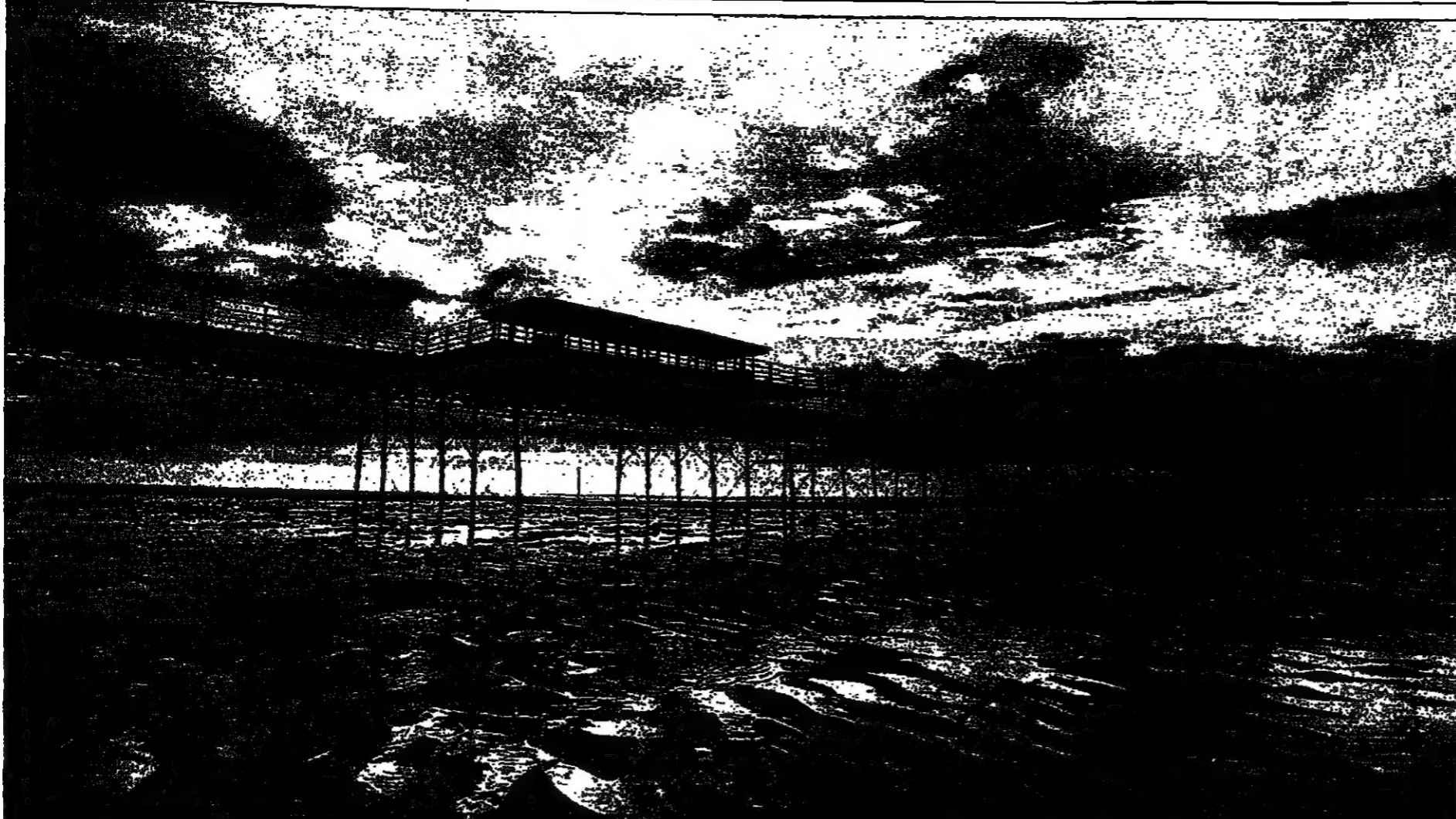
RUST and rot are threatening Southport Pier (above), the second longest in Britain and the inspiration for dozens of Victorian cast-iron seaside fantasies. writes Maryn Halsall. The Grade II listed structure, which heralded the high watermark of seaside pier construction, faces demolition without significant lottery funding.
